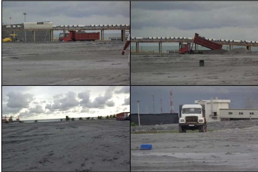
Picture/ Diagram No 06 - Bottom ash being deposited in the yard
