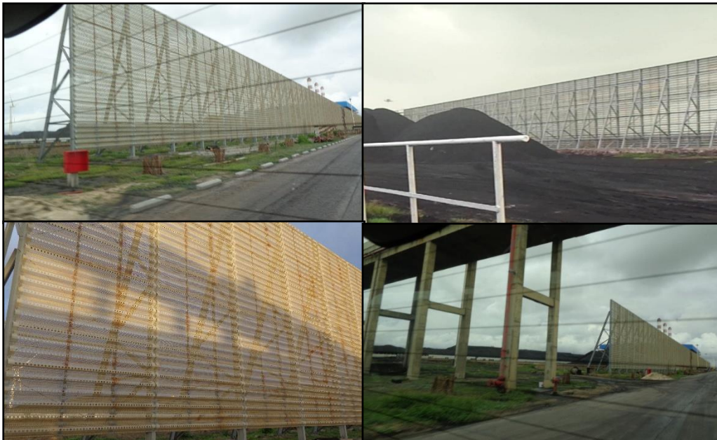
Picture/ Diagram No -09 Wind barrier existed around the coal yard
